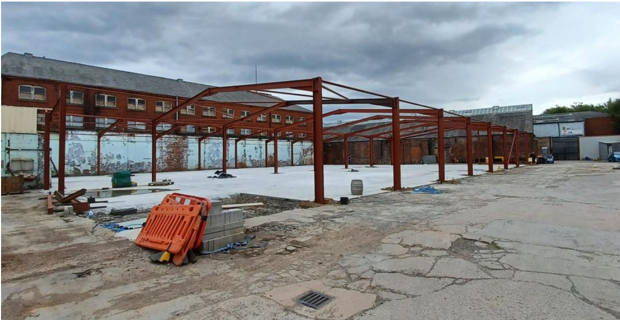
Photo 4: View of partially constructed building
