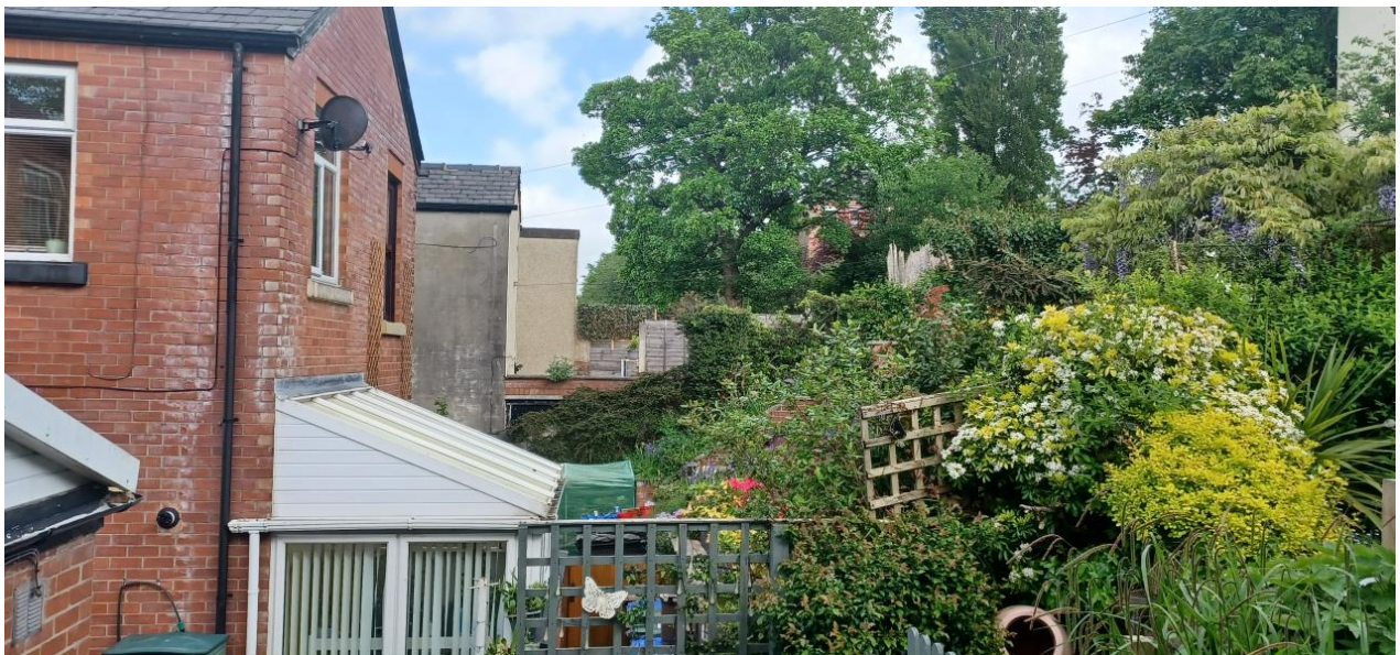
Photo 5: Change in levels to no.136 Mottram Road
